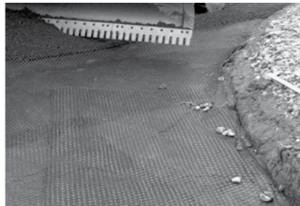
IMAGE 5: Placing Geogrid to accommodate curves.
