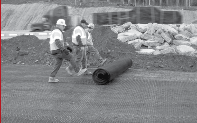
IMAGE 3: Rolling out Tensor® Geogrid.
