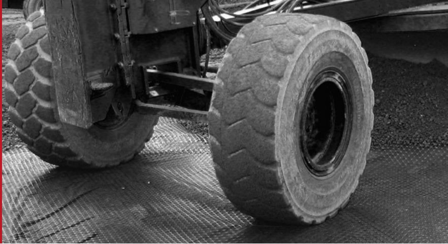
Geogrid can be trafficked directly by rubber-tired equipment. Refer to your local Tensar distributor or Tensar office for project-specific guidance.
