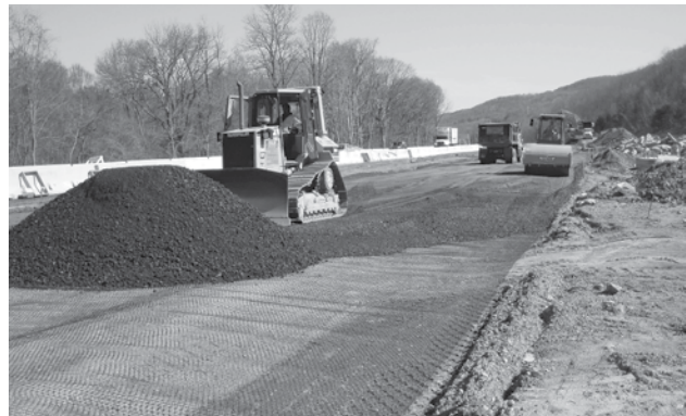
IMAGE 9B: Spreading aggregate fill over Tensor Geogrid.
