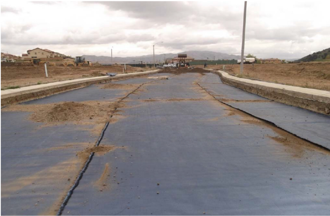
Figure 7(b): Photo of a Mirafi® H 2 Rx with geotextile edge terminated within.
