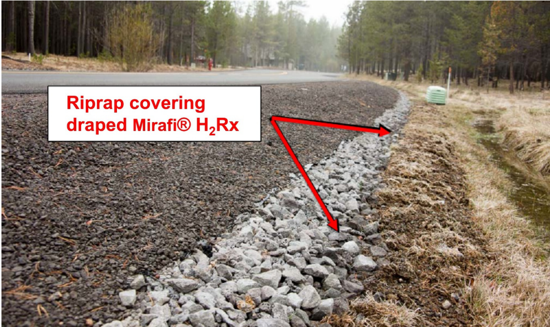
Figure 9(b): Photo of a Mirafi® H 2 Rx road project with draped geotextile tongue beneath a rock cover.
