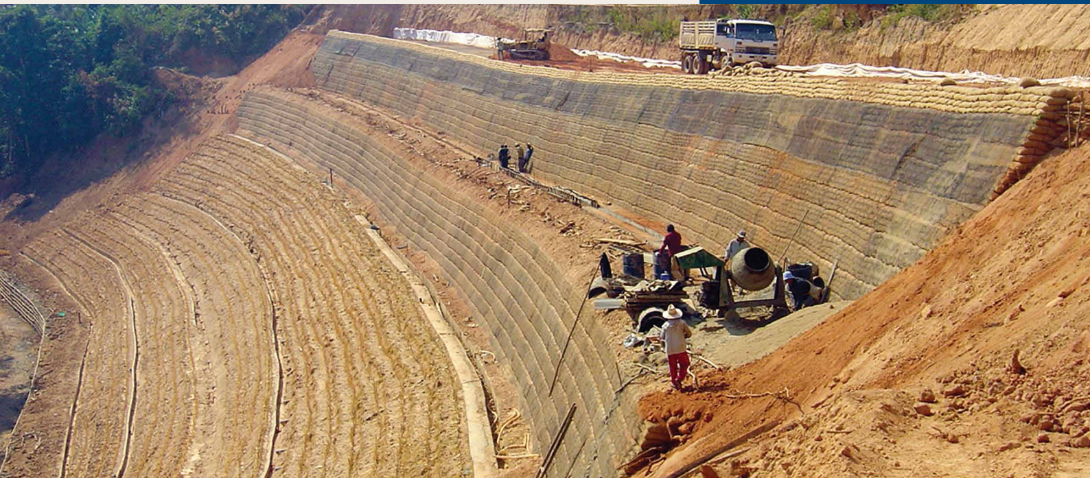
Miragrid® GX geogrids being wrapped around stacked geobags to construct a wall.
