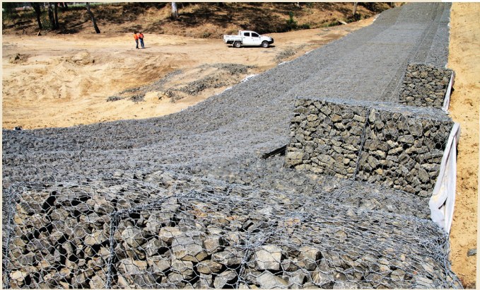
In total 162 Gabions over three sizes and 334 Reno Mattresses were installed
