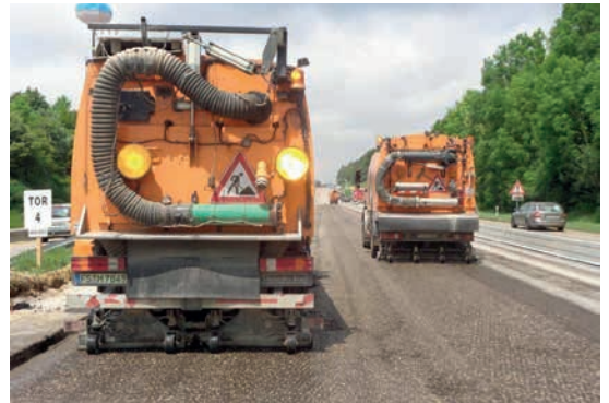
Pic. 1: Ultra High Pressure technology to clean the surface
