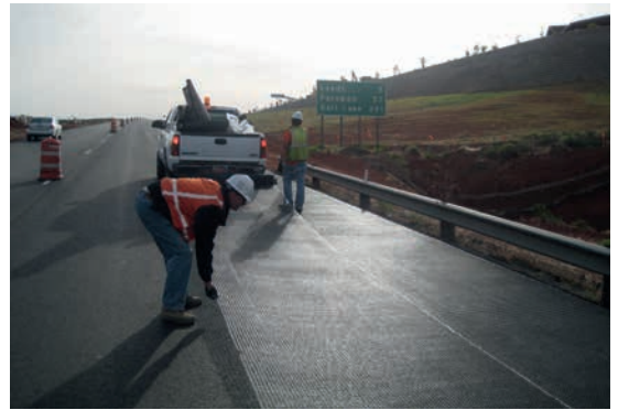
Pic. 4: Manual Installation of ADFORS GlasGrid
