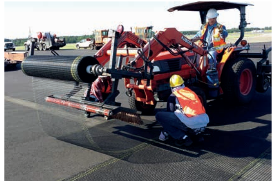
Pic. 3: Fabric Tractor Installation of ADFORS GlasGrid
