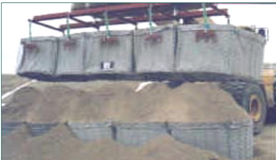
Figure 6: FLEXMAC® DT unit lifting operation
