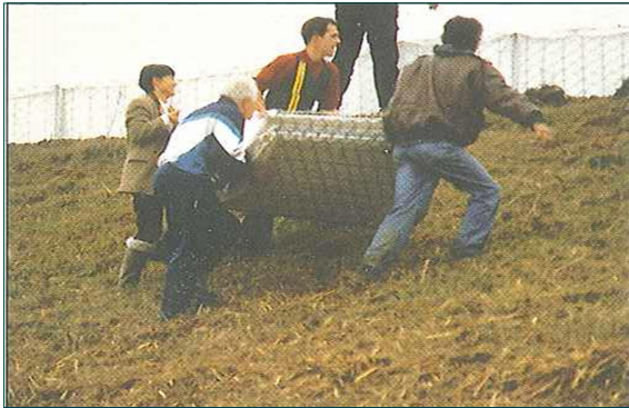
Figure 4: manual transportation of FLEXMAC® DT unit
