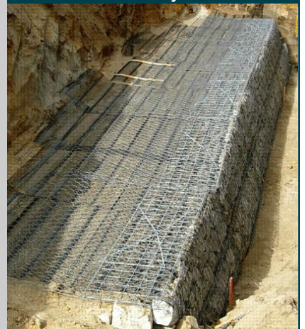
Green Terramesh Wall - New Zealand
